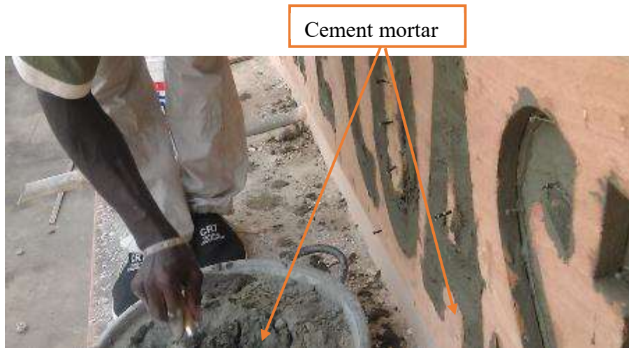
Figure 12: Filling the template (Mould) with mortar, Cape Coast Metropolitan Assembly, Cape Coast. by James Ekow Appiah, 2016.
