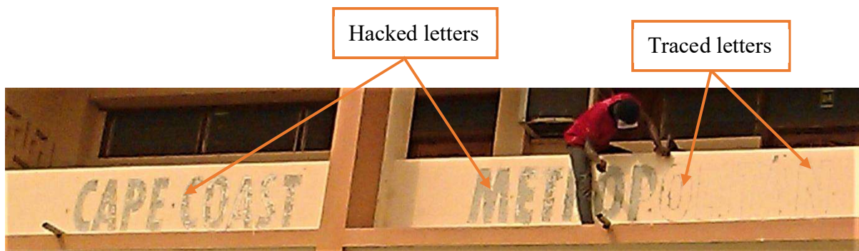
Figure 8: Tracing and hacking of letters on wall, Cape Coast Metropolitan Assembly, Cape Coast. by James Ekow Appiah, 2016.
